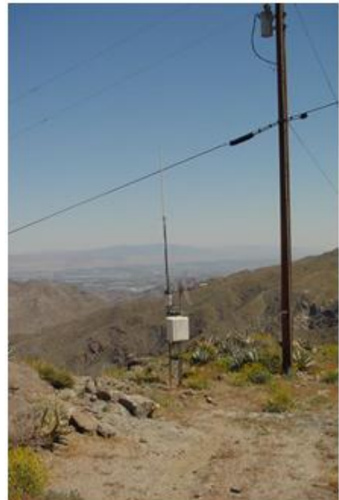
Photo 2-8 Existing HPWREN repeater tower and electric pole at Agave Hill site
