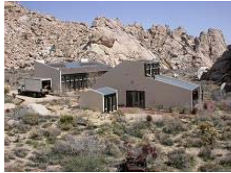
Photo 2-7 Allanson Administrative Building
