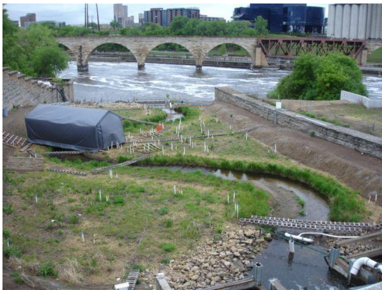
Photo 1-11 OSL, showing existing setup for instruments
