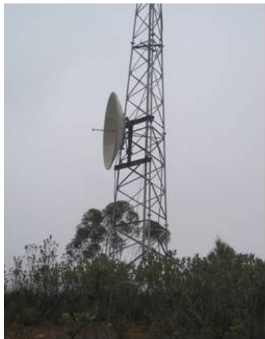
Photo 2-6 Existing tower at the Main Repeater Station site
