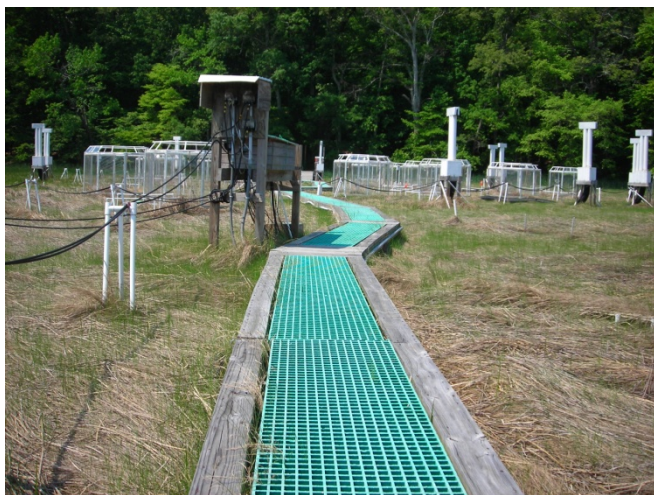
Photo 2-1 A recently rebuilt boardwalk at SERC: the proposed new boardwalks would be of similar construction
